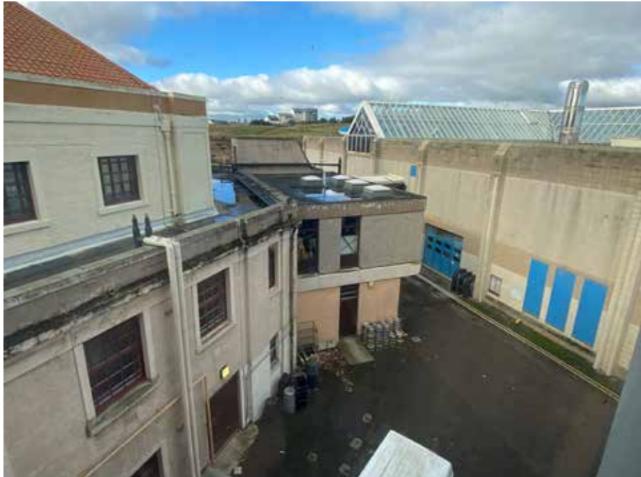
Poor quality extension to original building
