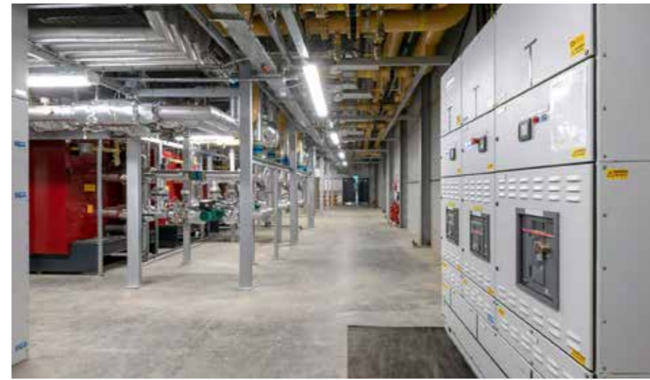
Interior Installation of TECA Energy Centre
