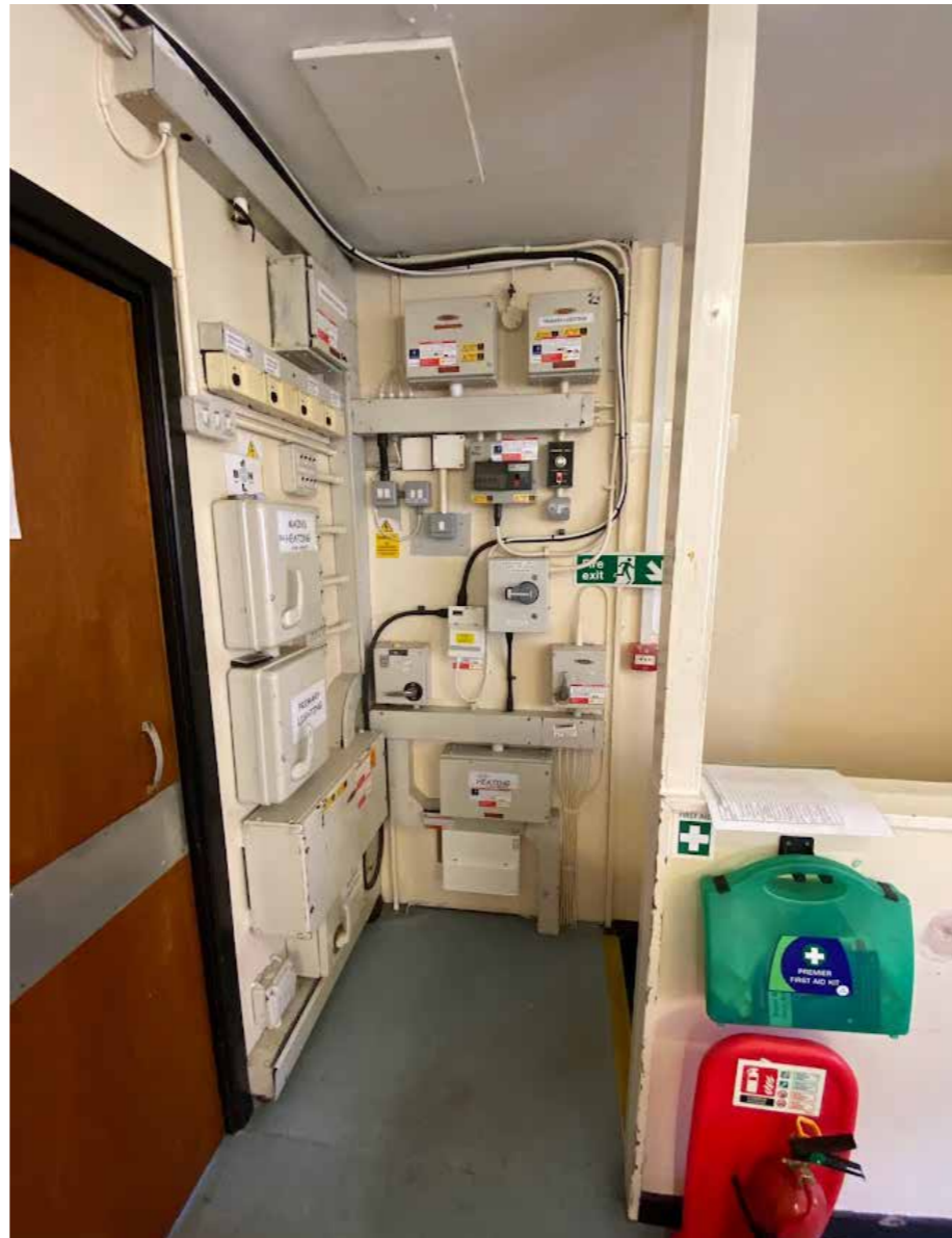
Unprotected escape staircase and exposed services
