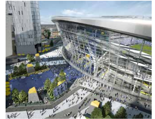
Integrated podium deck - Tottenham Hotspur Stadium
